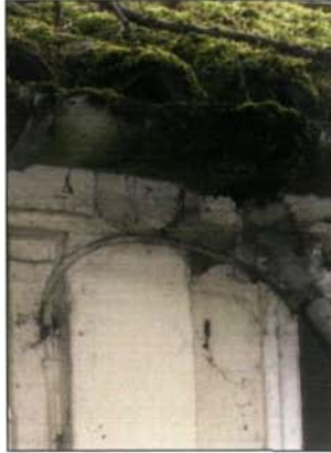
Moss and lichen growth on asbestos cement roofing and gutters
