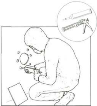
Attach the replacement panel with adhesive
