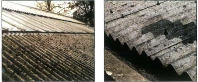
AC sheets used as roofing
