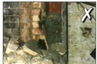
Broken asbestos insulating board, asbestos lagging and sprayed asbestos (limpet)
