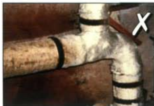
Broken asbestos insulating board, asbestos lagging and sprayed asbestos (limpet)
