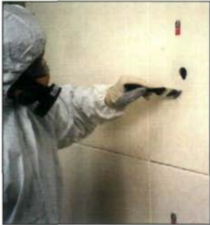
Seal the drilled edge with sealant
