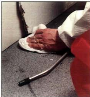
Wiping up debris with a damp rag
