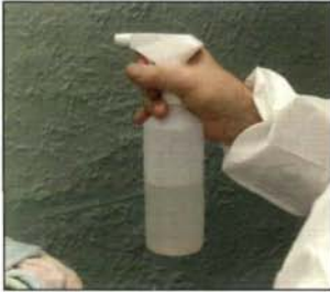
Spray at low pressure; high pressure spray could disturb fibres from asbestos paper under these tiles
