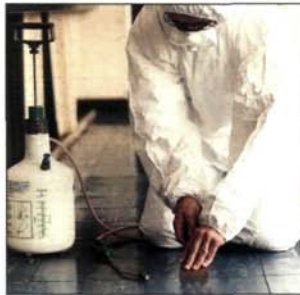
Spray water under the tiles to suppress dust as you lift them gently, avoiding breakage
