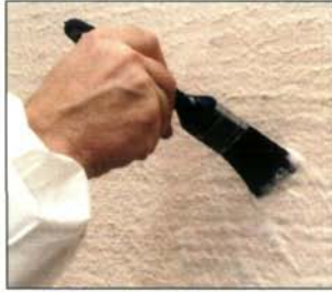
Sometimes it may be easier to wet the area using a brush or roller
