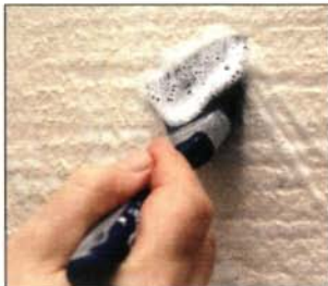
Paint sealant around the hole before you insert the screw. Use shadow vacuuming to control dust when removing screws
