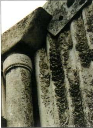
Moss and lichen growth on asbestos cement roofing and gutters
