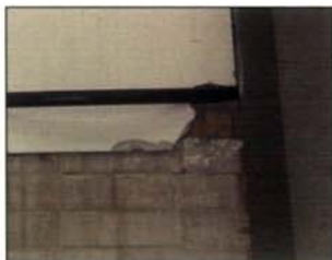
This damaged AIB needs to be covered and protected from further damage
