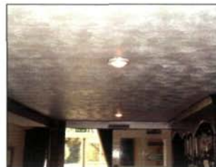
Textured coating is common on ceilings
