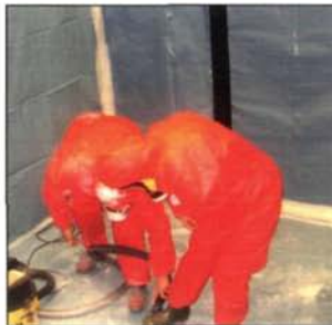
'Buddy' cleaning using a Class H vacuum cleaner
