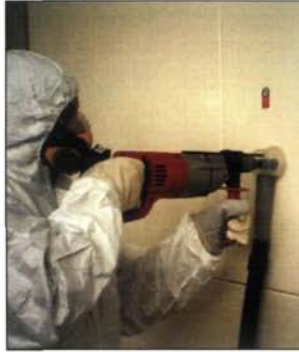
Control measures: Shadow vacuuming and plastic enclosures used as local extraction
