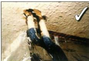
Damaged textured coating, asbestos cement roofing and an asbestos-containing gasket
