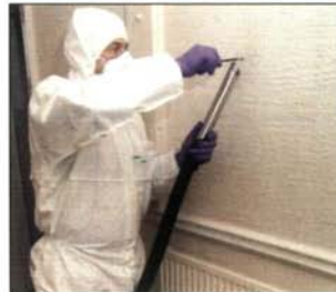
Paint sealant around the hole before you insert the screw. Use shadow vacuuming to control dust when removing screws
