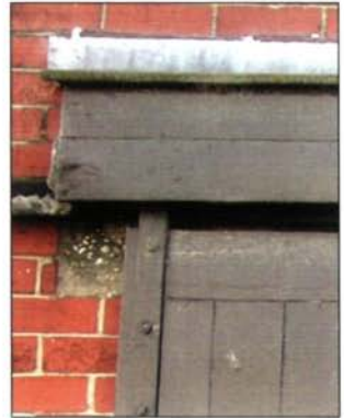
Built up bituminous roofing and bituminous asbestos fabric over a doorway
