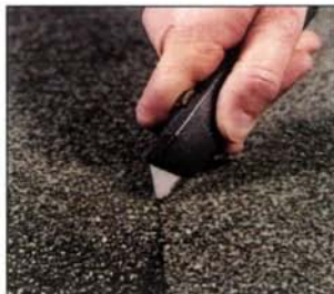
Cut and remove manageable sections
