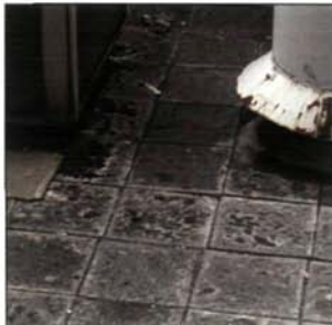
Asbestos cement tiles on a roof
