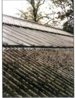
Moss and lichen growth on asbestos cement roofing and gutters
