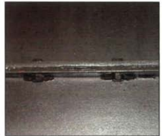
String gasket between metal sheets
