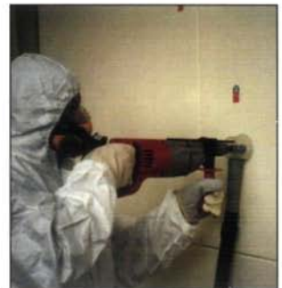
Control measures: Shadow vacuuming and using plastic enclosures as local extraction
