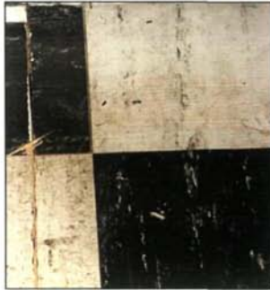
Floor tiles that contain asbestos can also have asbestos-paper backing, or be fixed with asbestos-containing mastic
