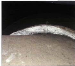
Joint packing on a flue
