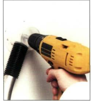
Control measures: Shadow vacuuming and plastic enclosures used as local extraction
