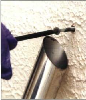
Control measures: Shadow vacuuming and plastic enclosures used as local extraction
