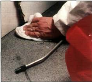
Wipe up dust and debris with a damp rag
