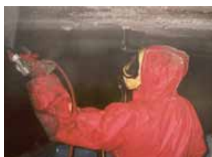
Figure 1.6 Controlled removal of asbestos
