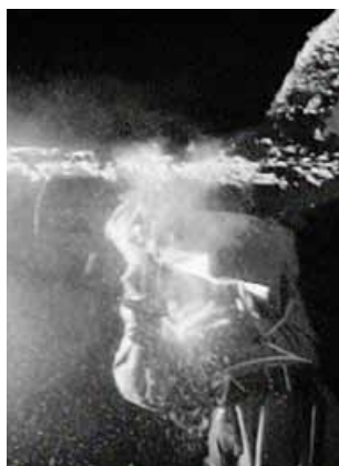
Figure 7.1 Uncontrolled dry stripping
