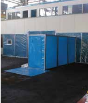
Figure 6.1 Enclosure with three-stage airlock
