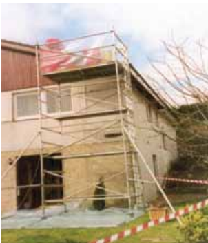
Figure 6.2 Work without an enclosure
