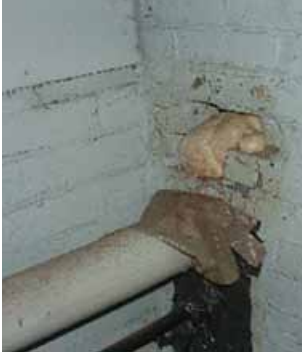
Figure 6.4 An enclosure sealed with expanding foam
