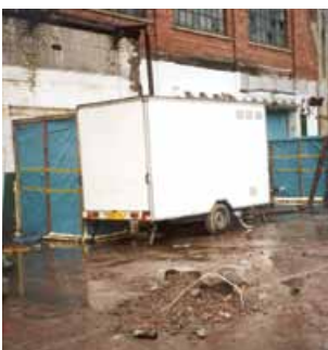
Figure 6.6 DCU attached directly to an enclosure
