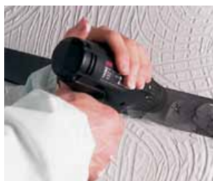
Figure 7.7 Textured coating being drilled through paste
