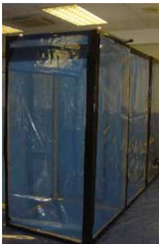
Figure 6.12 Flap arrangements for airlocks
