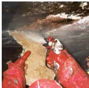
Figure 7.15 Spraying thin coating
