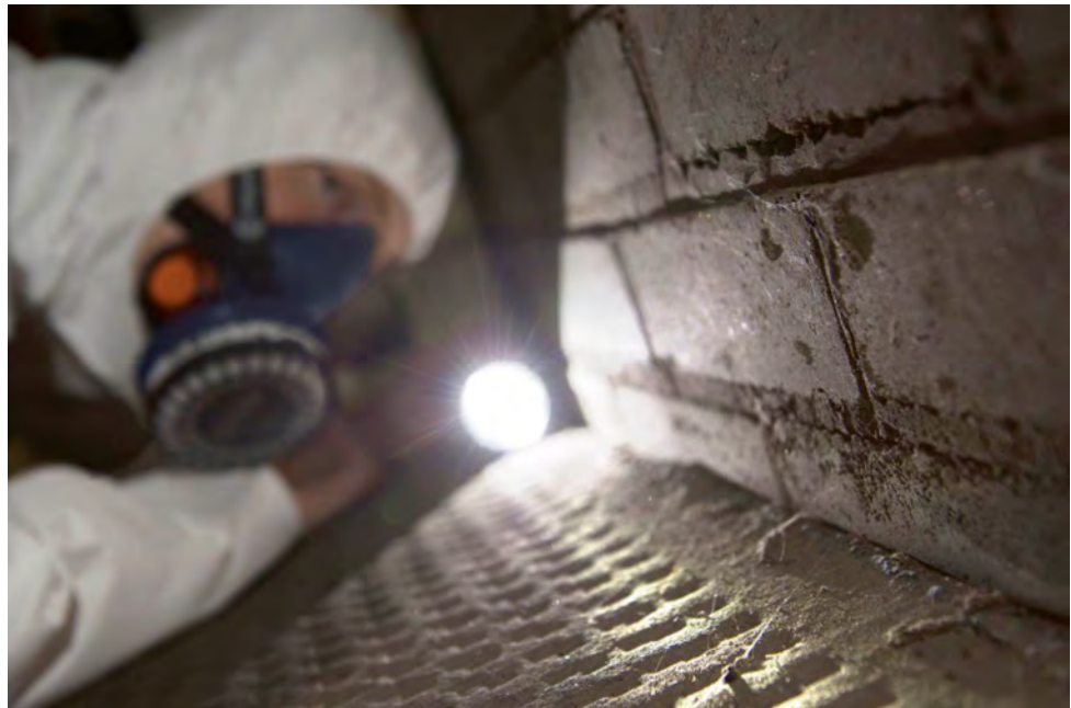
Figure 6.2 Analyst carrying out a detailed visual inspection
