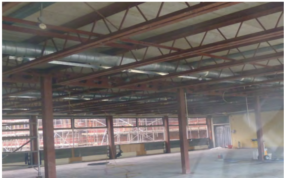
Figure 4.4 Photograph of a site where dust is likely to be present on high-level surfaces
